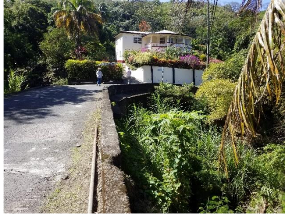
Figure 12.15: Gouyave to Florida road (looking east towards site F)
