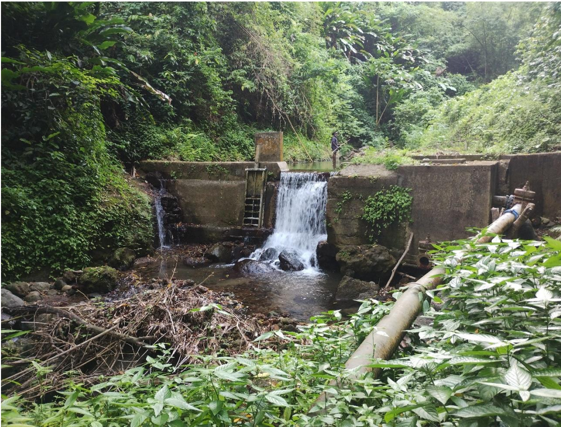
Figure 3.2: Mt. Reuil dam and water intake
