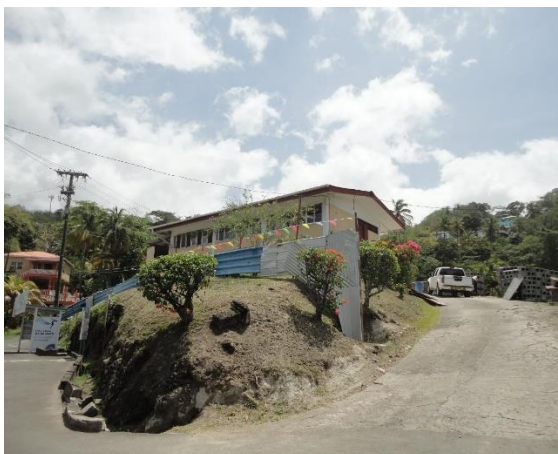
Figure 12.12: Settlement of Mt Rich (view uphill north towards site C)
