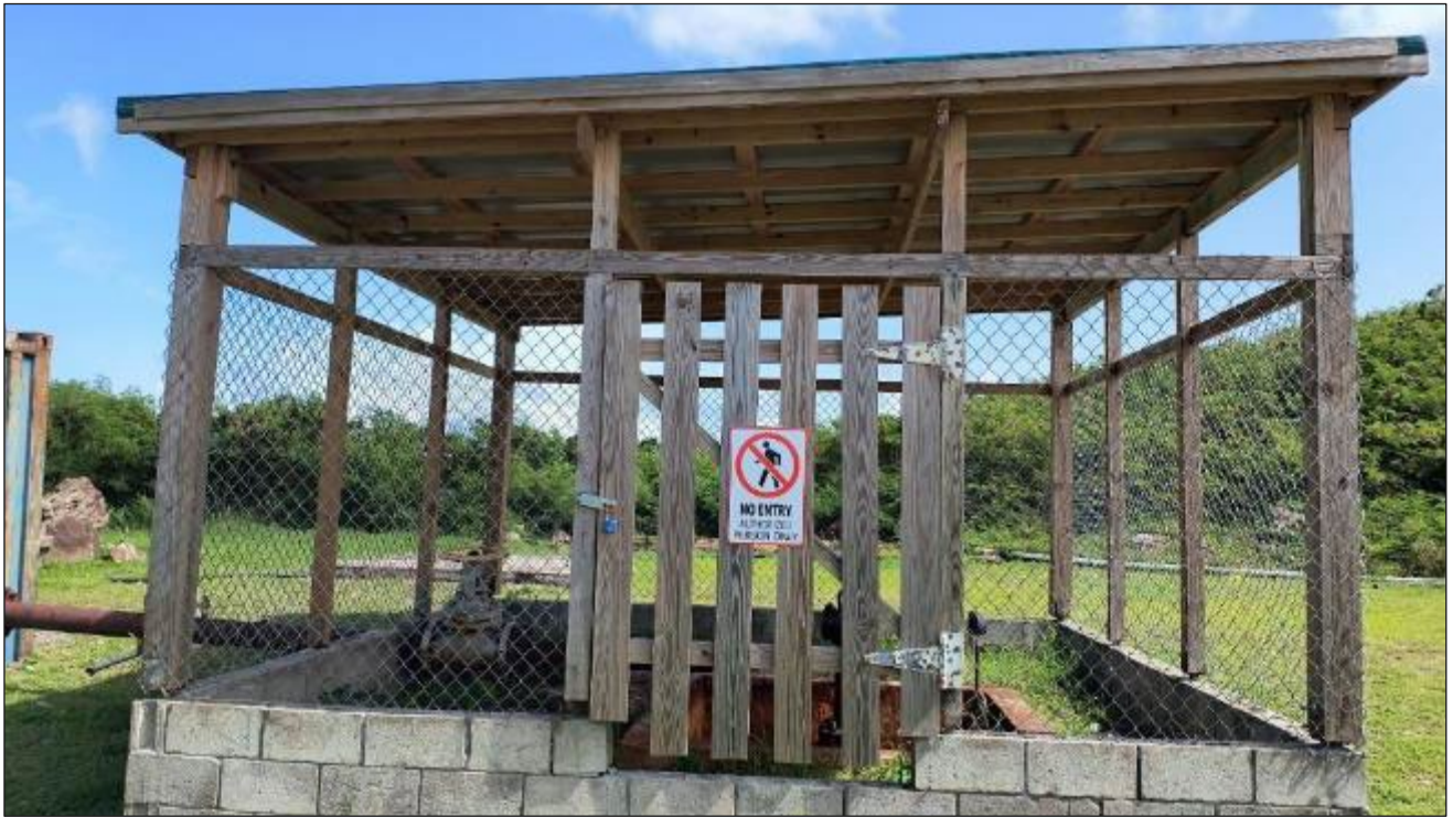
Photo 9: Well pad area / N-4 barricaded.
