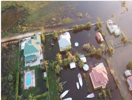
Inundated homes at Western Pines
