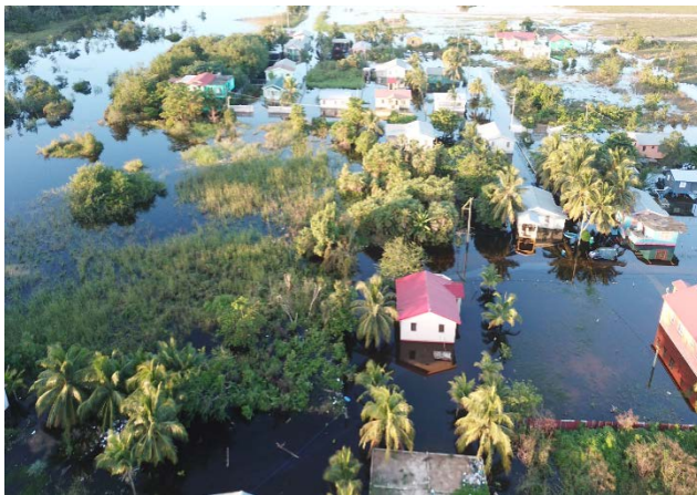
Fig 6: Inundated homes at Western Pine
