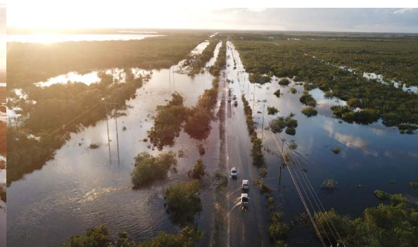
Fig 9: GP highway and west inundation
