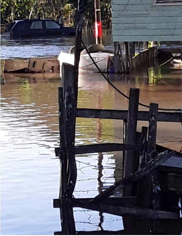
Residence being affected in the village of Lemonal
