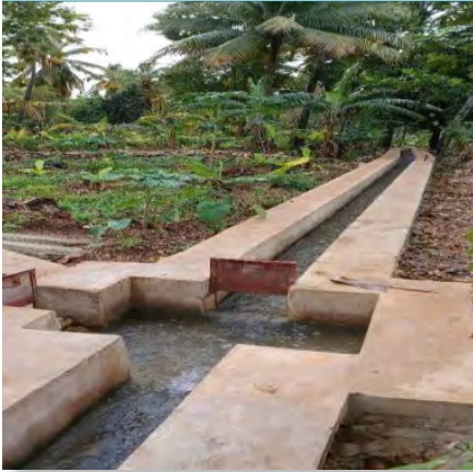
Newly Constructed Irrigation Canals
