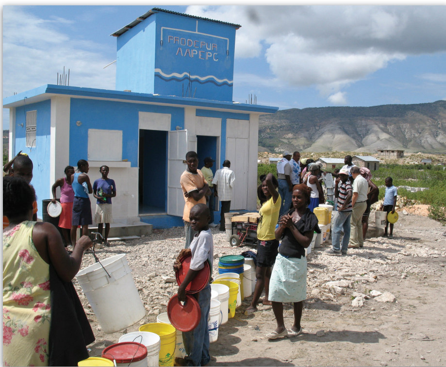
Potable water supply system in Haiti.
