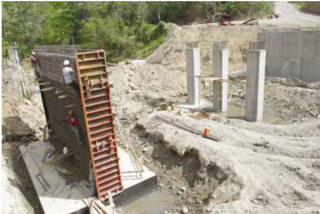
ST. LUCIA Large bridge construction under the CDB funded Roads Development Programme.
