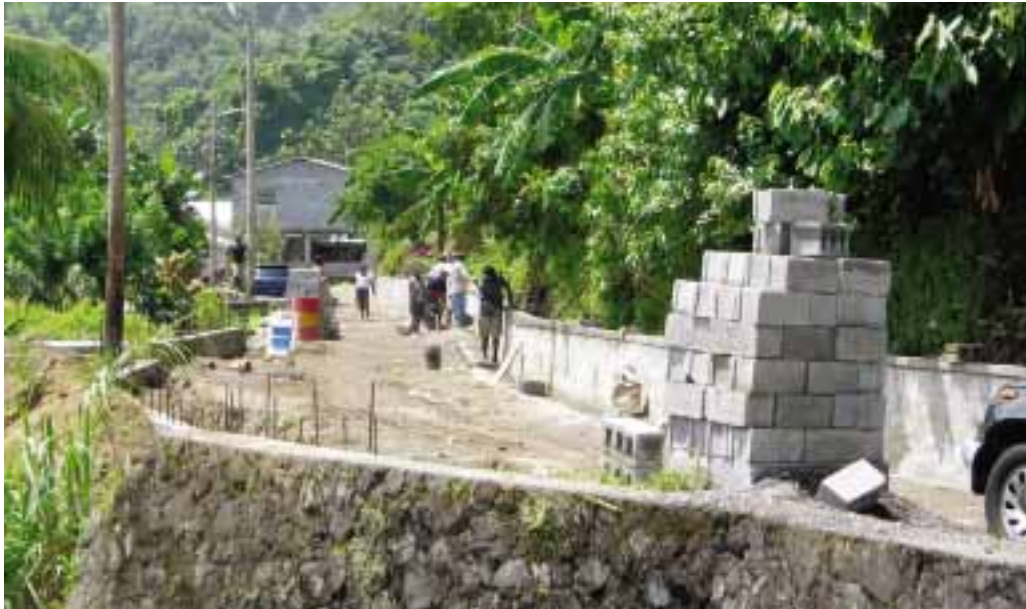
ST. VINCENT Community access at Galbar Road in Chateau Bel Air will be improved under BNTF 5.
