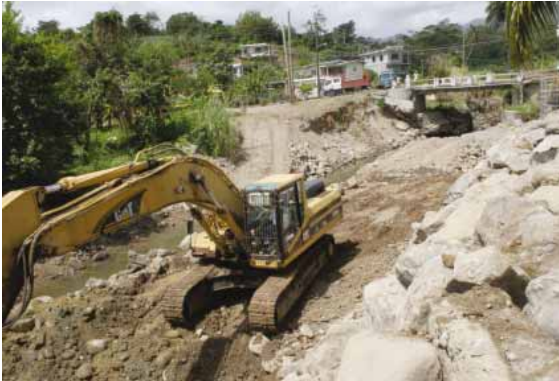
GRENADA CDB assisted the Government of Grenada in financing the reconstruction of approximately 2.1 kilometres of main arterial road and three bridges.
