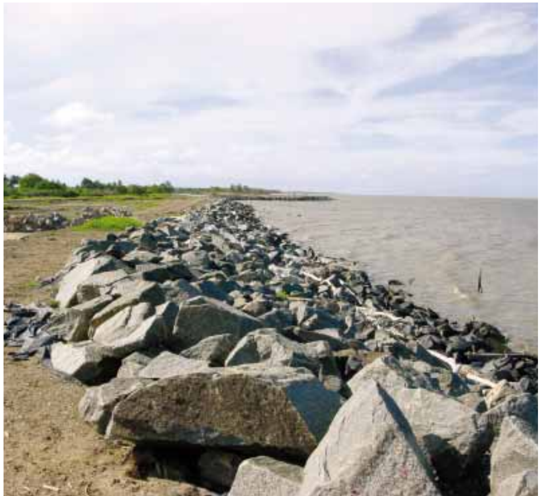
GUYANA The CDB has assisted the Government of Guyana emergency restoration of sea defenses. The project is designed to reconstruct the sea dyke and façade drain to prevent further salt intrusion and flooding in the West Berbice area.
