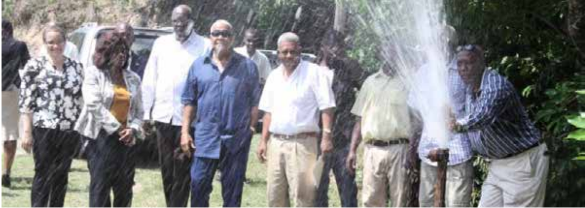
Site Supervisor of JSIF, Neville Williams turns on a pipe following the handing over ceremony for the commissioning of a water supply and booster station and tank in Thornton, St. Thomas. Sharing the moment are (L-R) JSIF Project Manager, Celia Dillon; Managing Director, Scarlett Gillings; Minister of Health, Fenton Ferguson; Minister of Water Land, Environment and Climate Change, Robert Pickersgill and Second Vice President of the St. Thomas Association of Branches, Rupert Scott.
