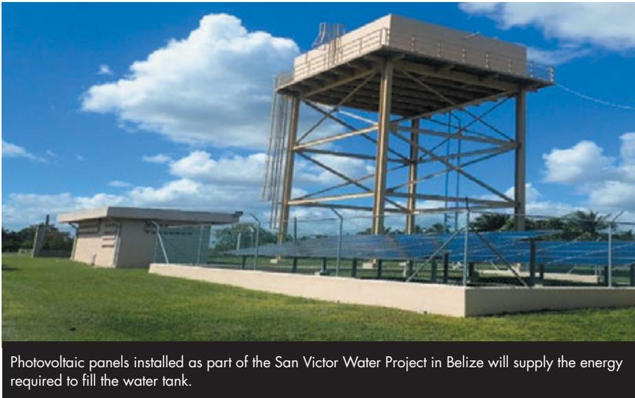
Photovoltaic panels installed as part of the San Victor Water Project in Belize will supply the energy required to fill the water tank.
