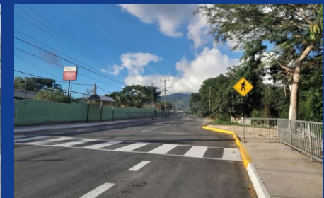
Upgraded Roadway Markings and Signage
