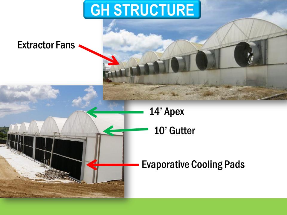
**Polycarbonate GH STRUCTURE Polytunnel Film Bracing to** withstand 150 mph winds **Bird Proof Netting**
