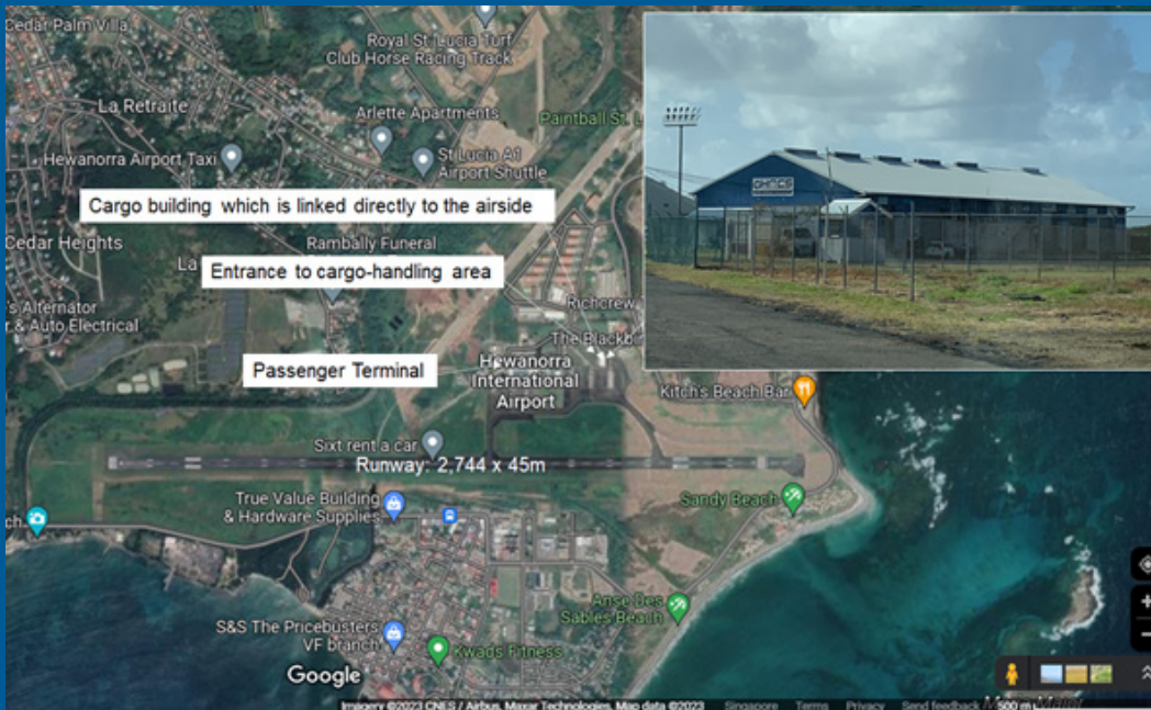
Figure 17: Cargo-Handling Facility at Hewanorra International Airport
