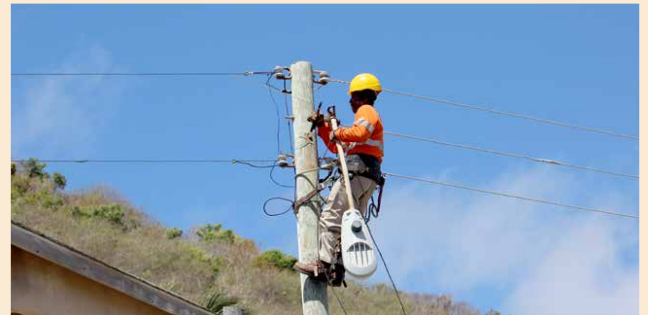
Before: A staff member from the St. Kitts Electricity Company installing LED lights as part of the CDB-funded Street and Flood Light Retrofitting Project.
