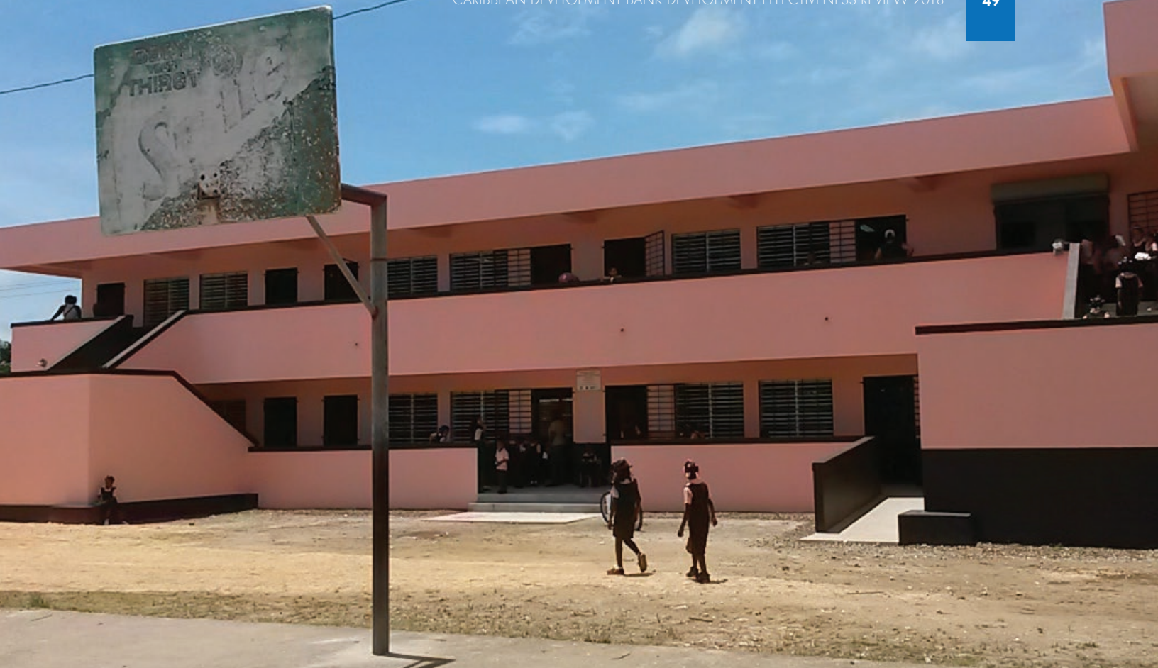
The newly constructed two-story classroom block at the Queen Square Primary School in Belize, which was financed under the Belize Social Investment Fund II Project. The new classrooms offer an improved learning environment for students in the Belize City District.
