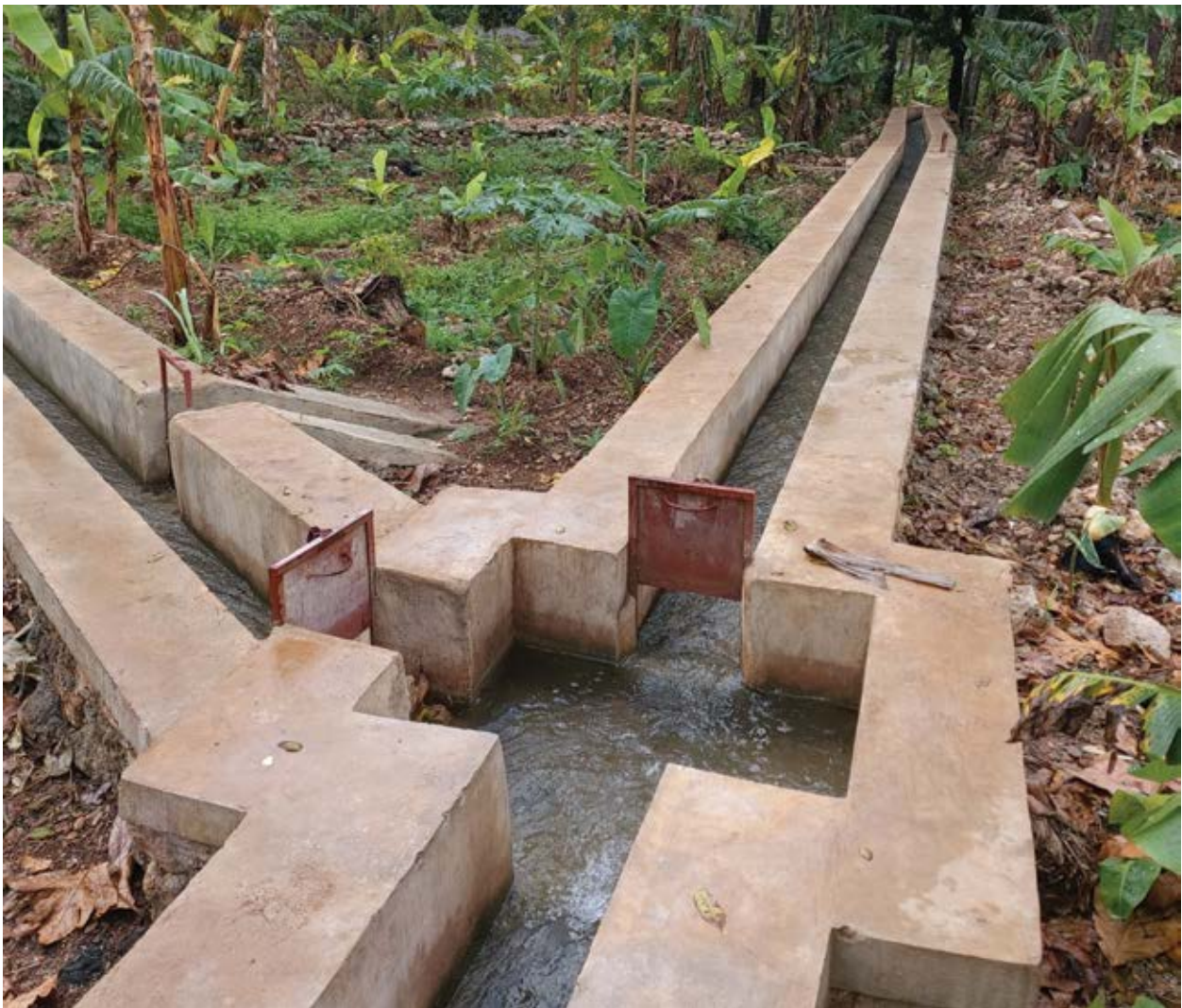
Distribution basin headwater channel and Augustave channel (Irrigated scheme, Lavalatière, Haiti)
