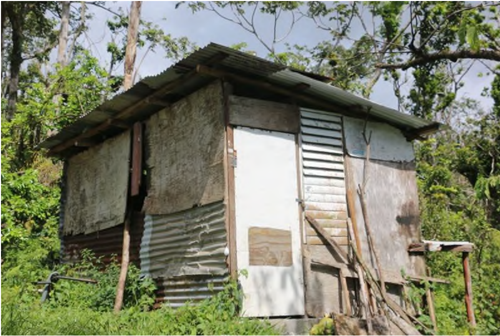
Figure B.5 : Shed C3
