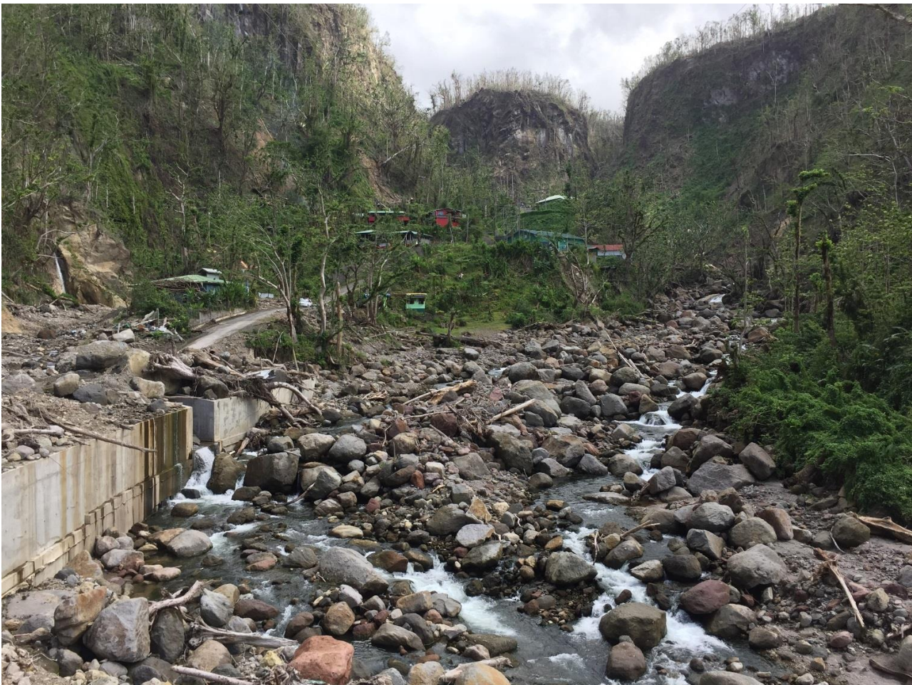
Figure 3.37 : The devastation caused by Hurricane Maria in the Roseau Valley
