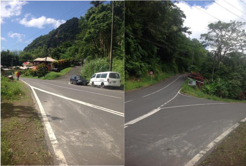
Figure 3.31 : Valley Road junction with the local road to Wotton Waven (looking north and south) (Source: Jacobs, 2016)
