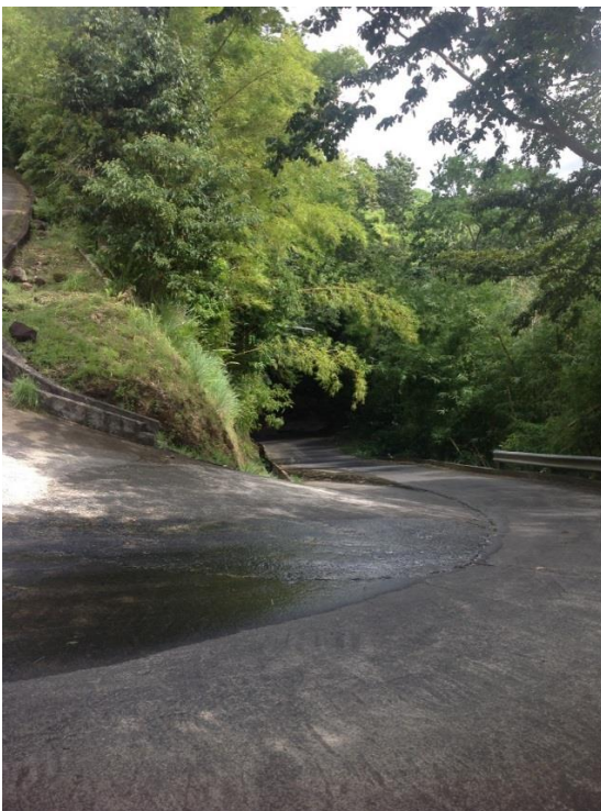
Figure 3.30 : Section of road that has been widened (Source: Jacobs, 2016).
