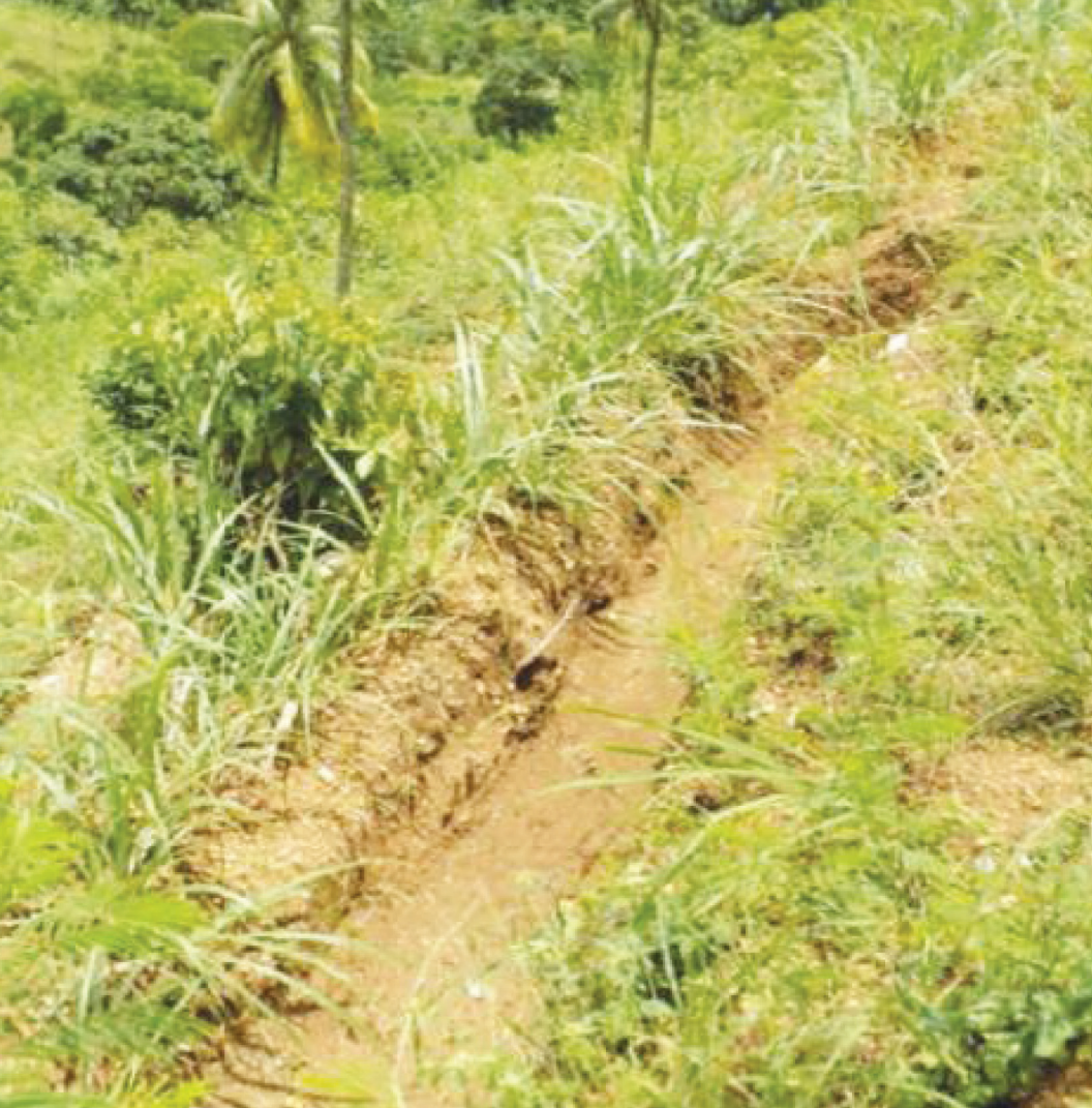
Diversion ditch - one of the methods used by farmers to reduce flooding risk.
