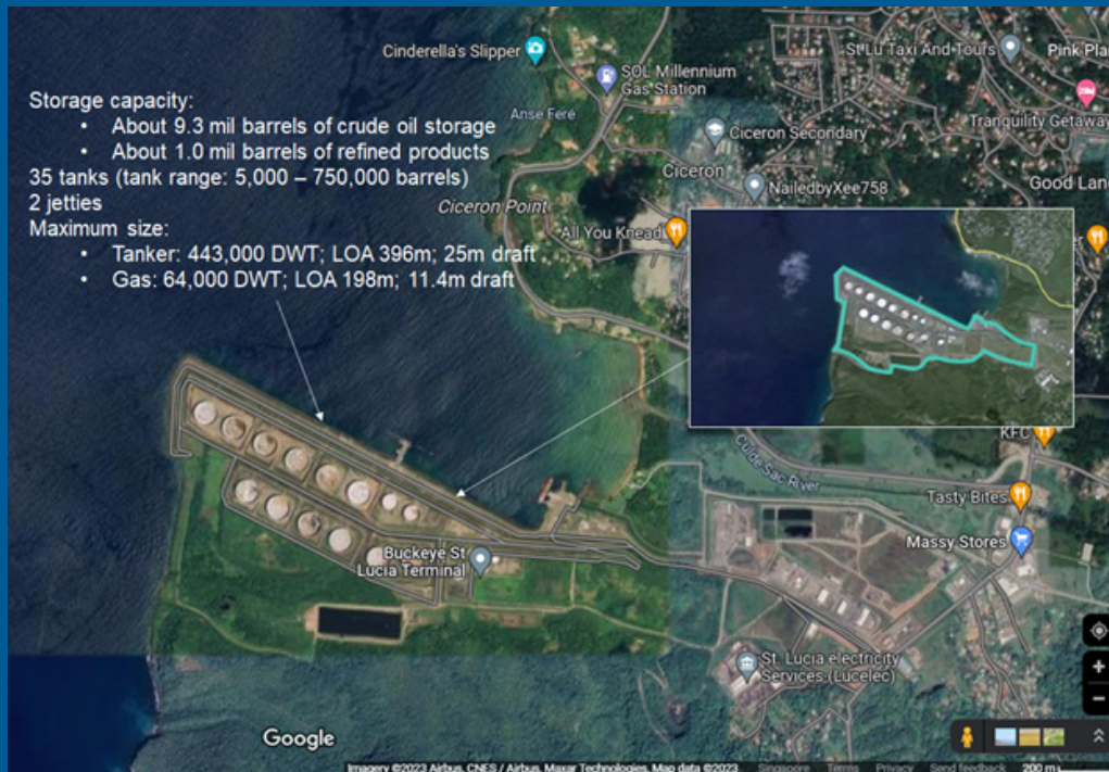
Figure 16: Buckeye Saint Lucia Terminal at Cul de Sac
