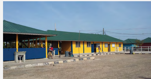
Dyke Road Fishing Complex, Jamaica: Built as part of Highway 2000, to relocate fisher folk who had been illegally occupying lands adjacent to the new Highway, as part of the project’s social responsibility programme.
