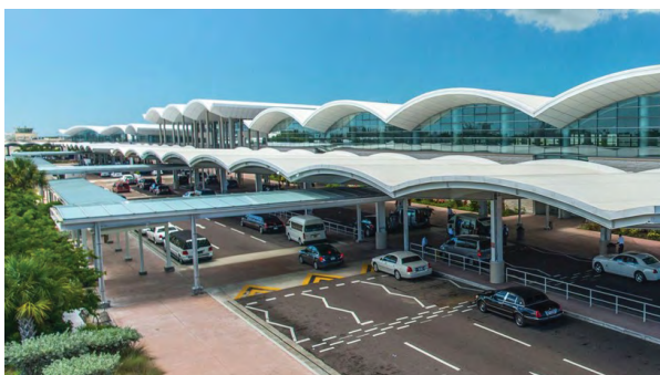
Linden Pindling International Airport, Nassau, Bahamas: A 10-year management contract with YVR Airport Services Ltd. (YVRAS) to manage, operate and redevelop the airport.
