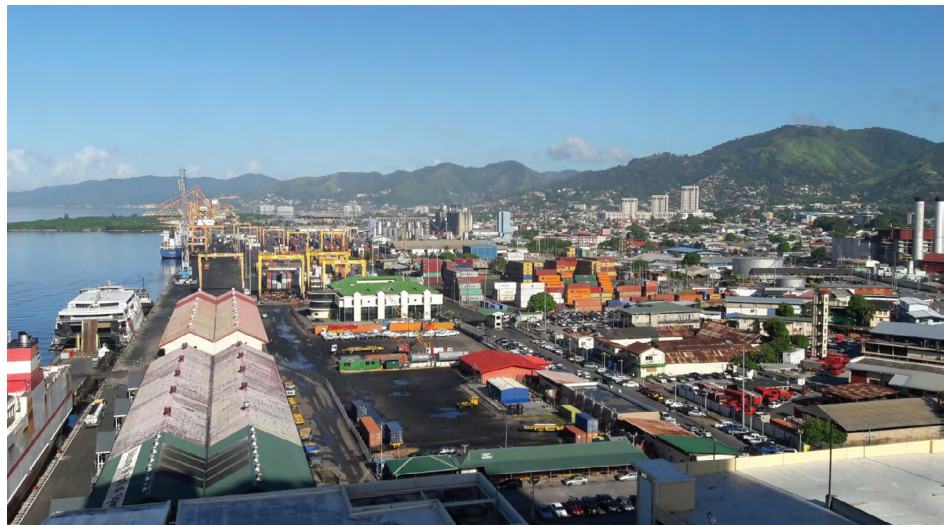
Container Port of Port of Spain, Trinidad and Tobago. PPPs can be used to improve the capacity and efficiency of the Region's ports.
