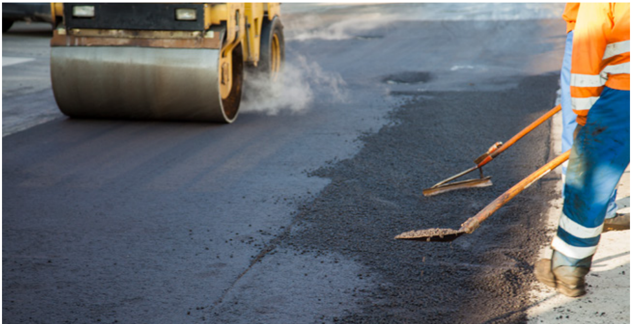
Laying new layer of asphalt
