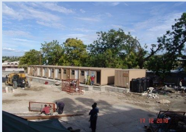
New Temporary Offices under construction for GOH agencies within the Ministry of Public Works, Transport and Communications
