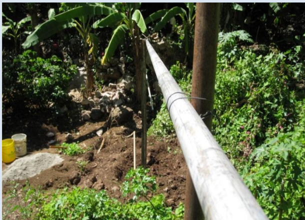
Small Scale Irrigation project
