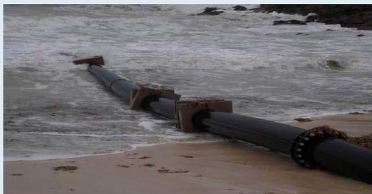
**APUA RO intake line: concrete anchors shifted and line displaced.**
