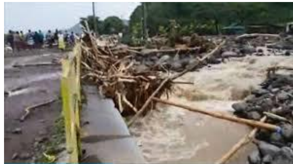
Photo 1.10. Bridge blocked by debris, Dominica, Tropical Storm Erika, 2015
