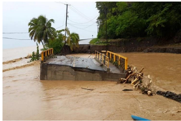
Photo 1.9. Coastal bridge abutments washed away, Dominica, Tropical Storm Erika, 2015
