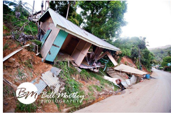
Photo 1.19. Landslide undermines house, Saint Lucia, Hurricane Tomas, 2015 (Source:
