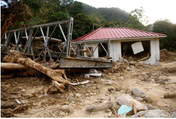
Photo 1.5. Impact of flooding during Hurricane Tomas, Saint Lucia, 2010
